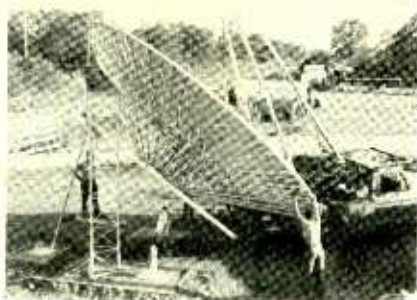
FIG. 1—SATELLITE RECEIVING ANTENNA as it is being installed on steel mounting posts.
